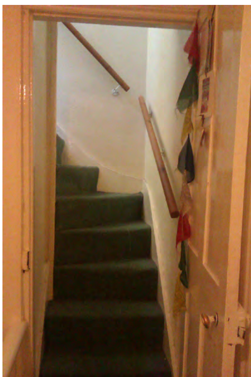
Figure 3: Photo of door
